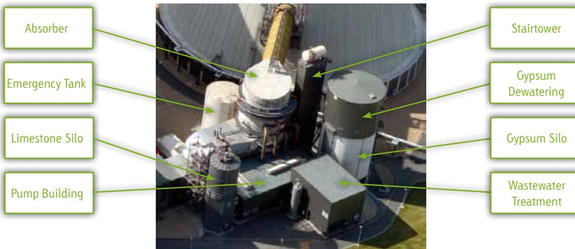
Figure 4: Wet Limestone FGD plant Lünen [Source Trianel]
